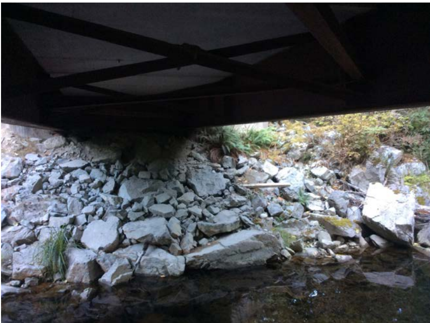
Right Bank Abutment when facing downstream
