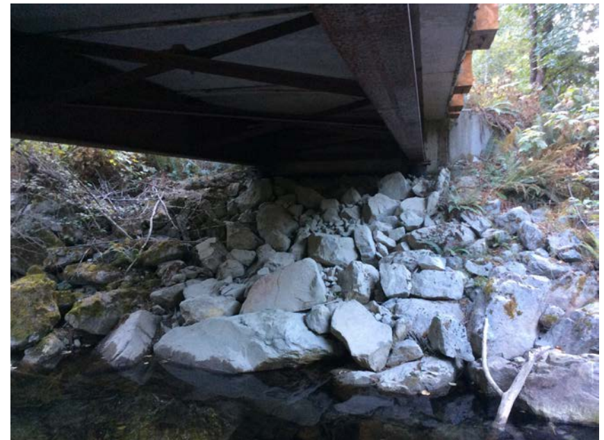
Left Bank Abutment when facing downstream
