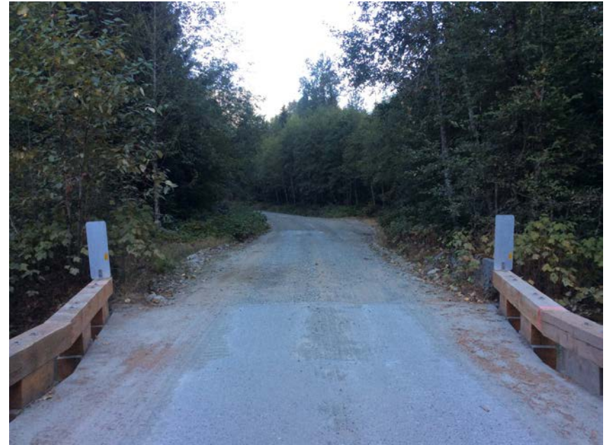
Right approach viewed from bridge
