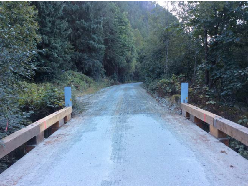
Left approach viewed from bridge
